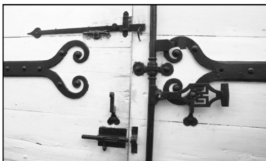
Medieval hinges hold the Maison de Quaker door. meeting in France.
